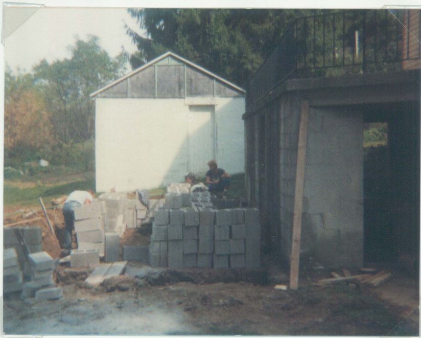
Adding second garage under porch. Old garage at rear taken down during development.
