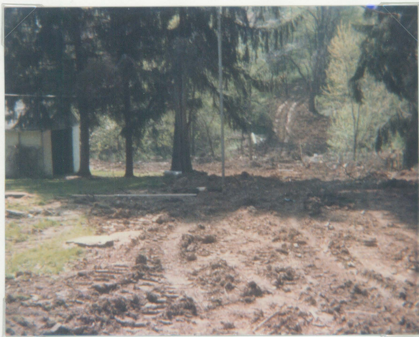
old garage back yard mud sewer pipe laid
