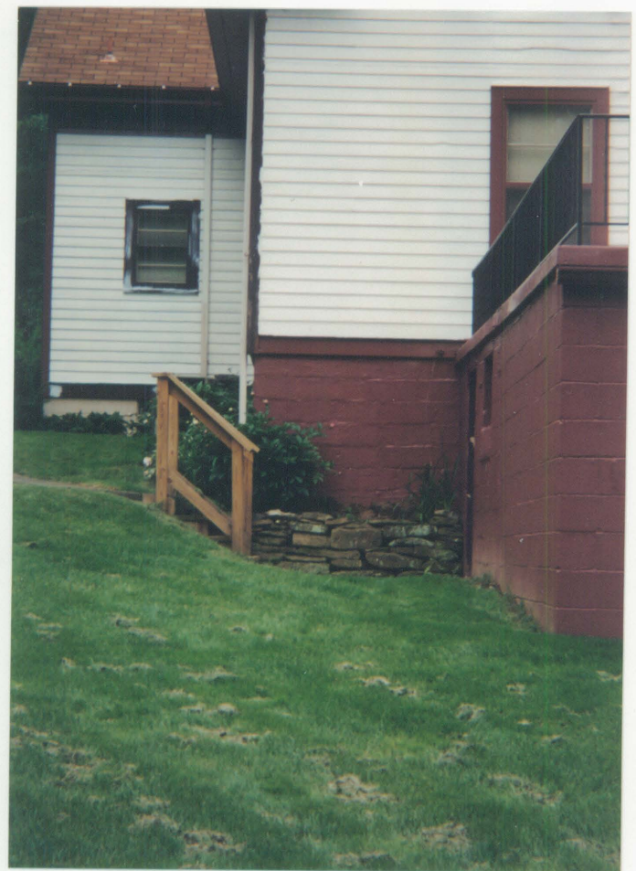
View from West - June, 1995 Painting in progress. New stairs to garage.
