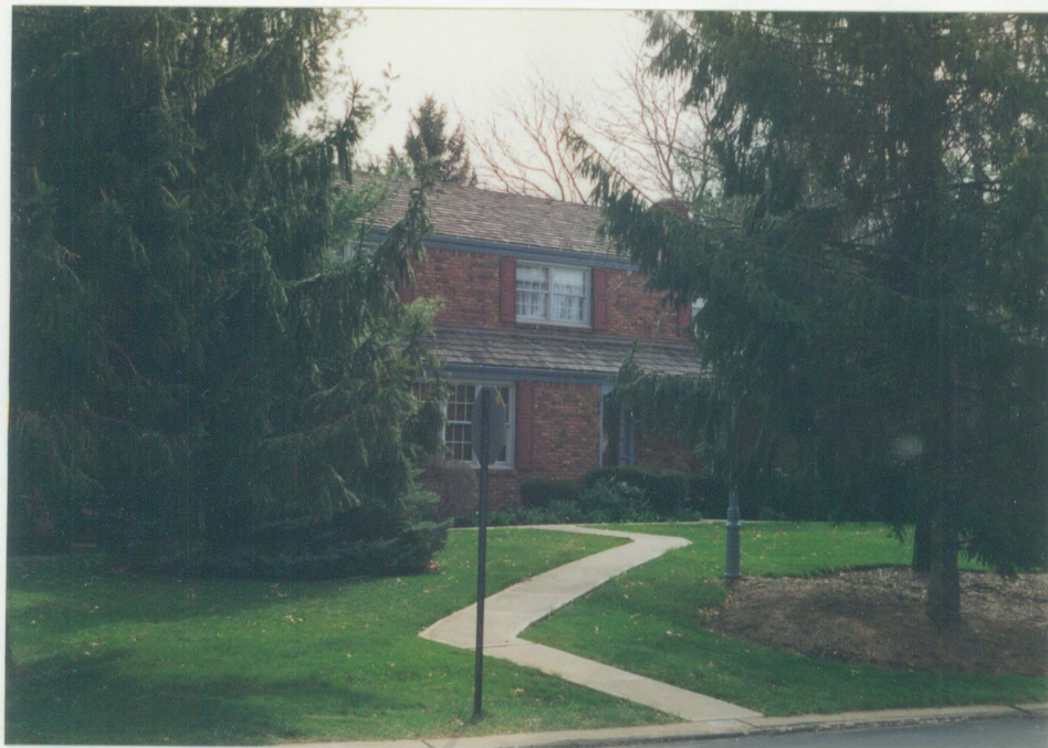
Degenhardt house - Boxer Height Developer
